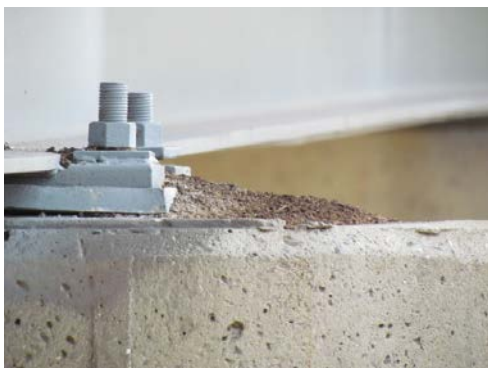
Photo 5: Guano deposit on pier, obscuring structural features.
